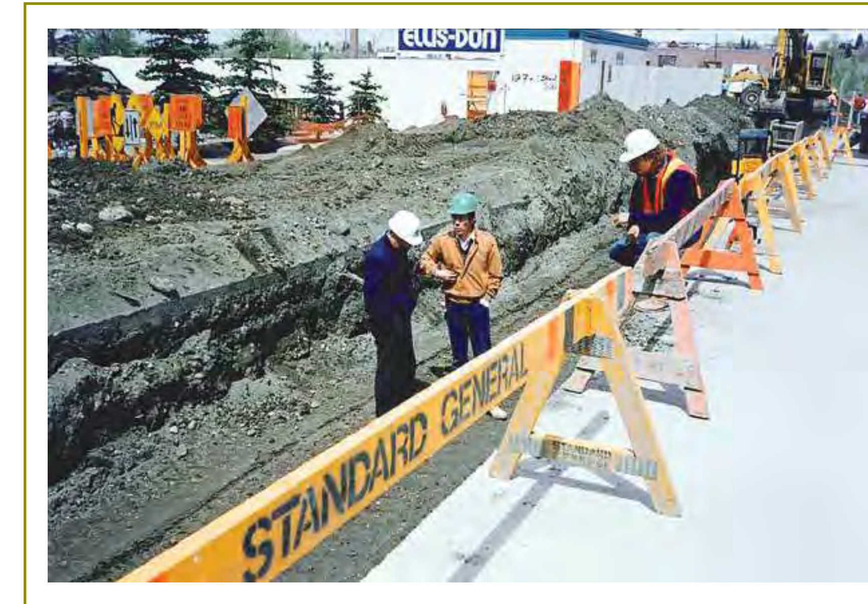
Construction Site for the Calgary Chinese Cultural Centre, 1991.
