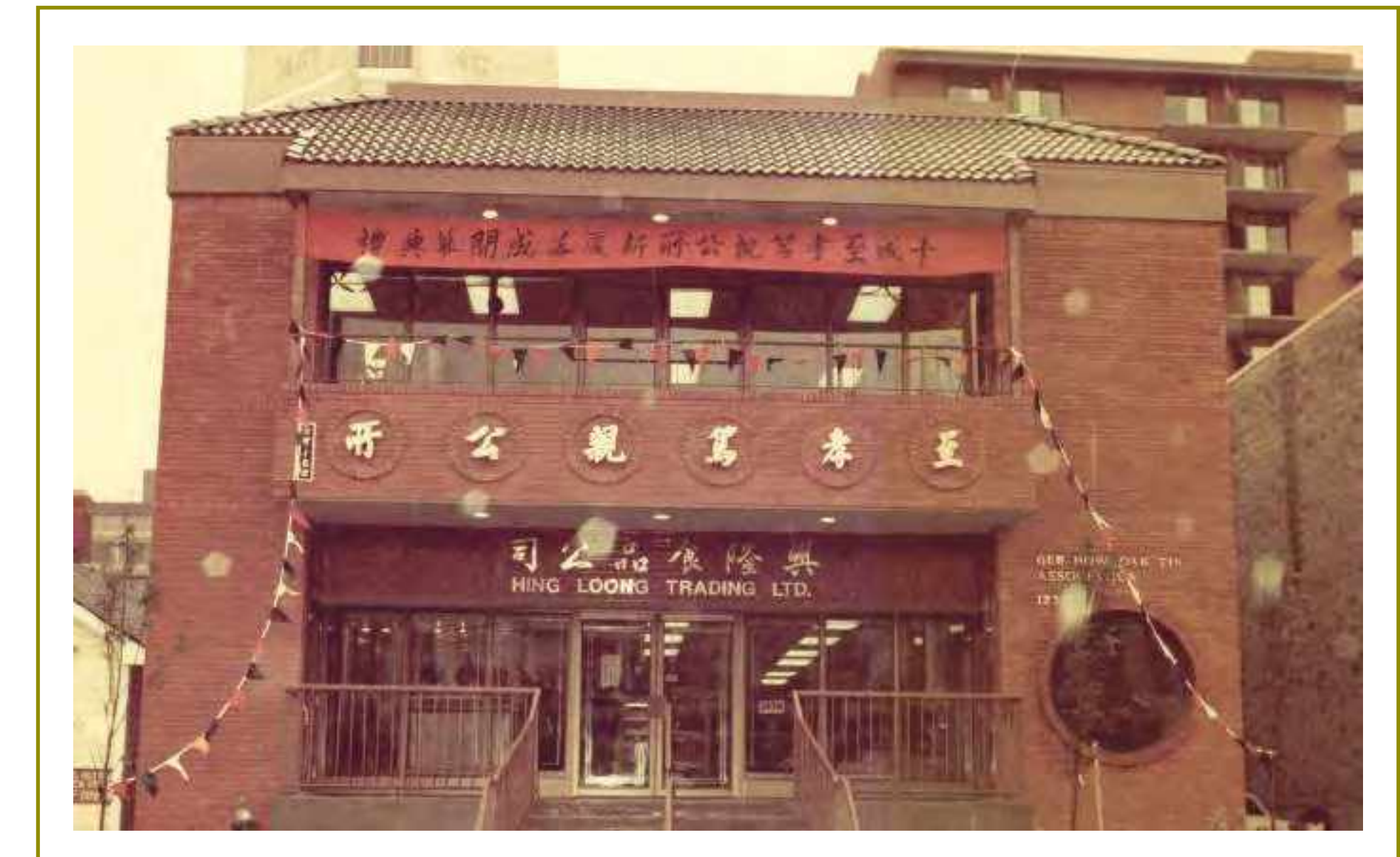
In 1982, a new building was constructed at the same location replaced the former one, and still continues to serve as the Calgary branch for the Gee How Oak Tin Benevolent Association today.
