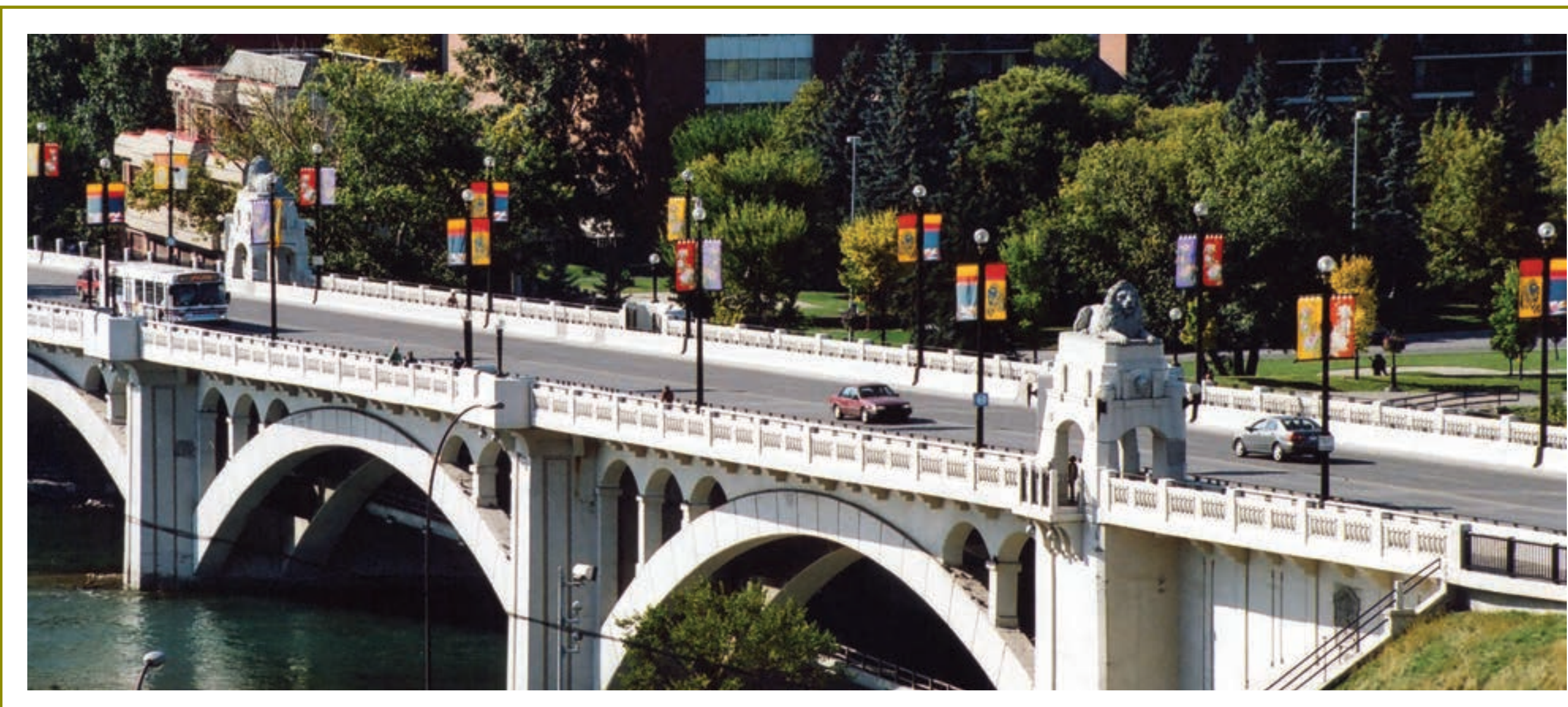
Centre Street Bridge, 2008.
