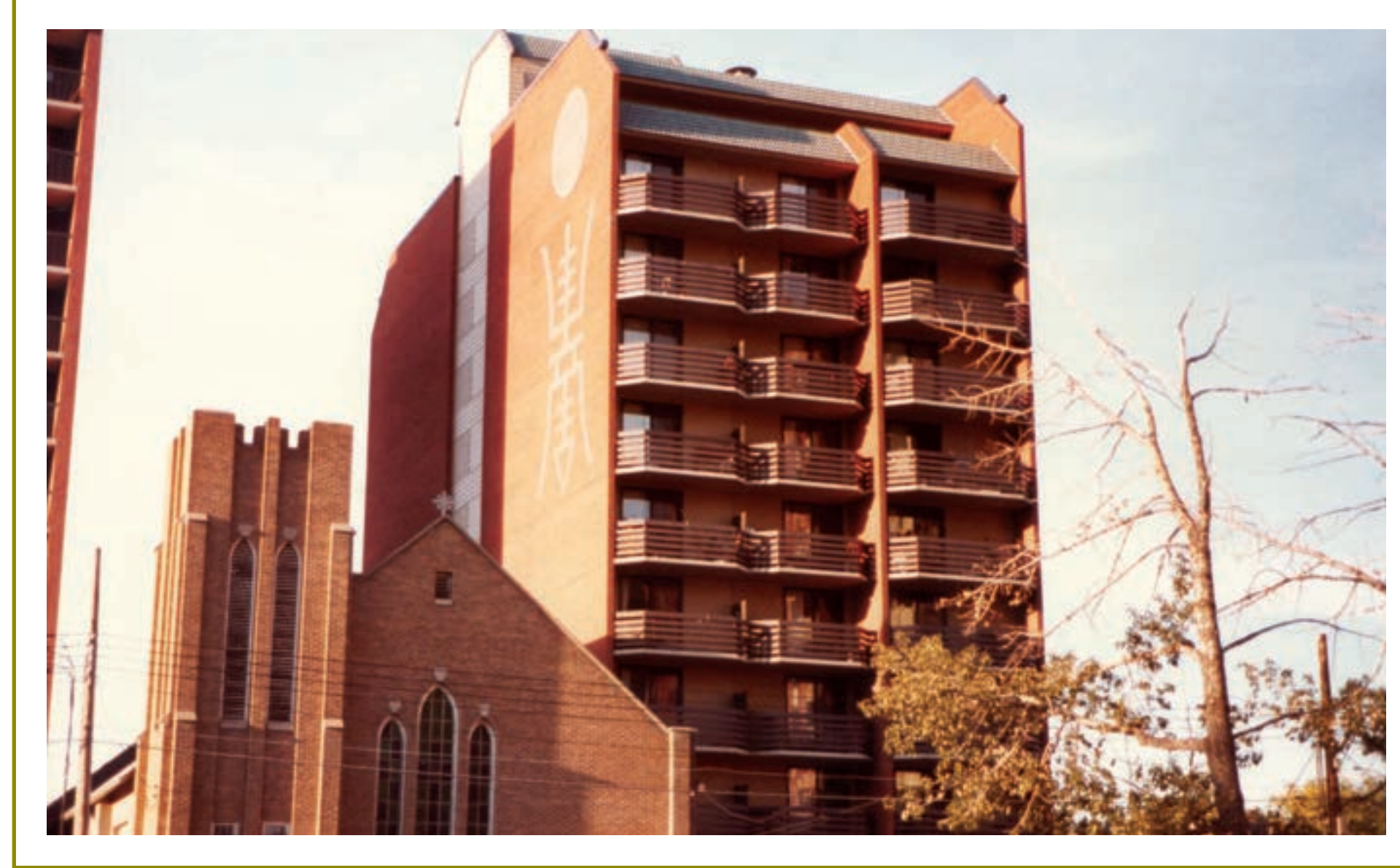
Oi Kwan Place Building, 120, 2nd Avenue SW, circa early 1980s.
