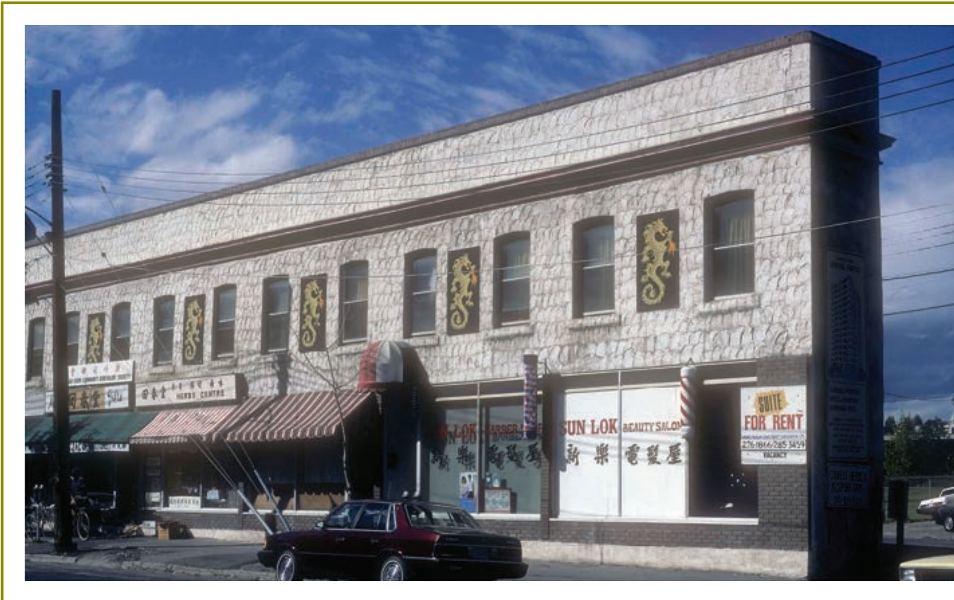
East End of Flat Iron Block, 128 2nd Avenue SE, 1986.
