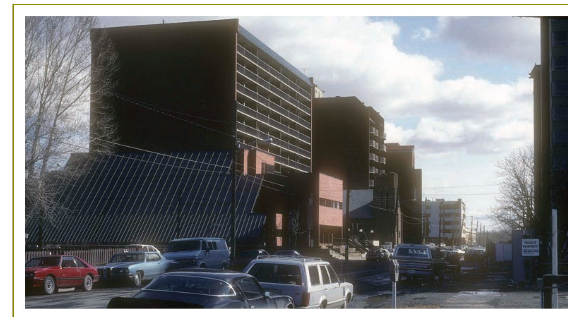
View east from 1st Street and 2nd Avenue SW, with Calgary Native Friendship Centre building at forefront, Bowside Manor behind, Chinese United Church and Oi Kwan Building, circa, 1980s.
