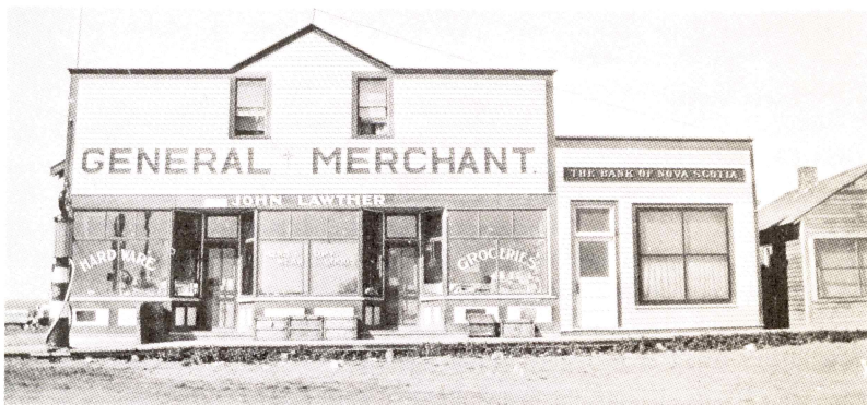
John Lawther's store at Queenstown.
