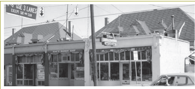
310, 310A and 312, Centre Street S, 1972.
