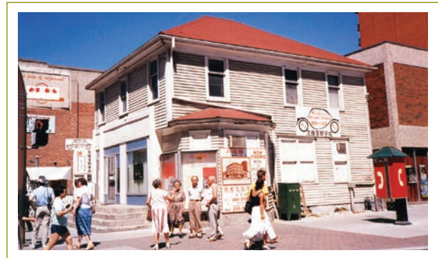
Dr. Chow's House, Centre Street and 3rd Avenue SE, 1988.
